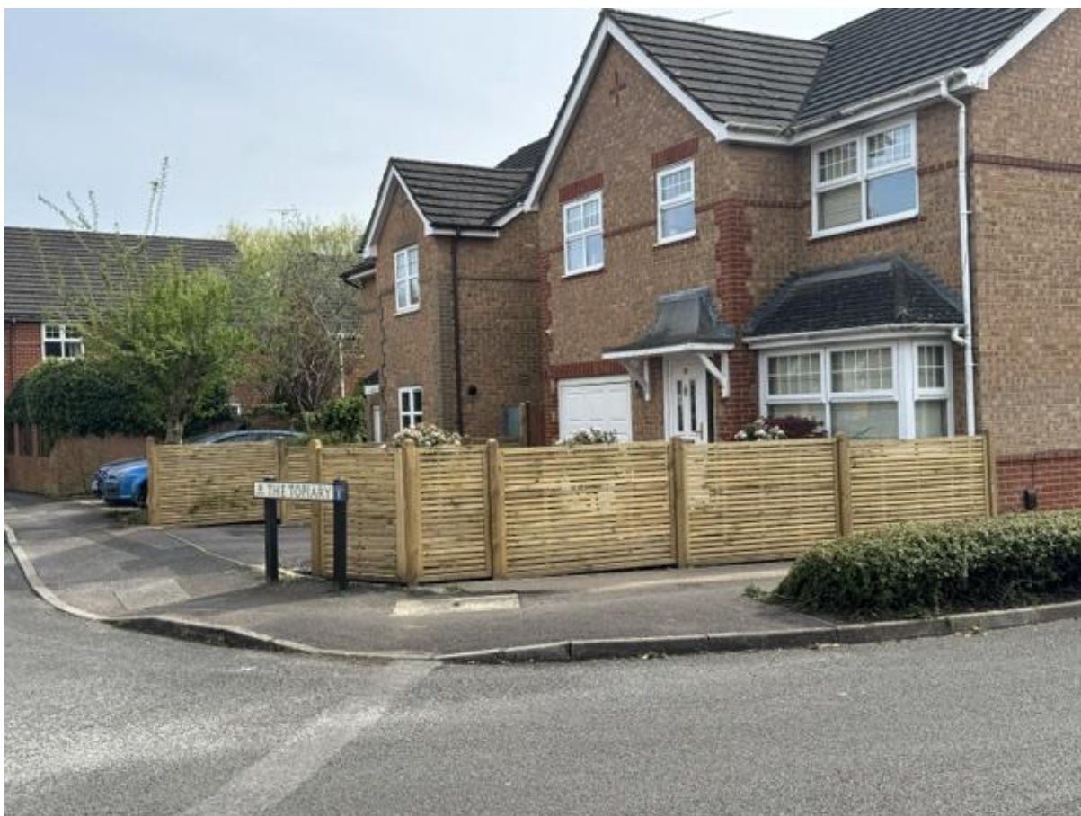
Figure 1 – view of fence at 28 The Topiary
