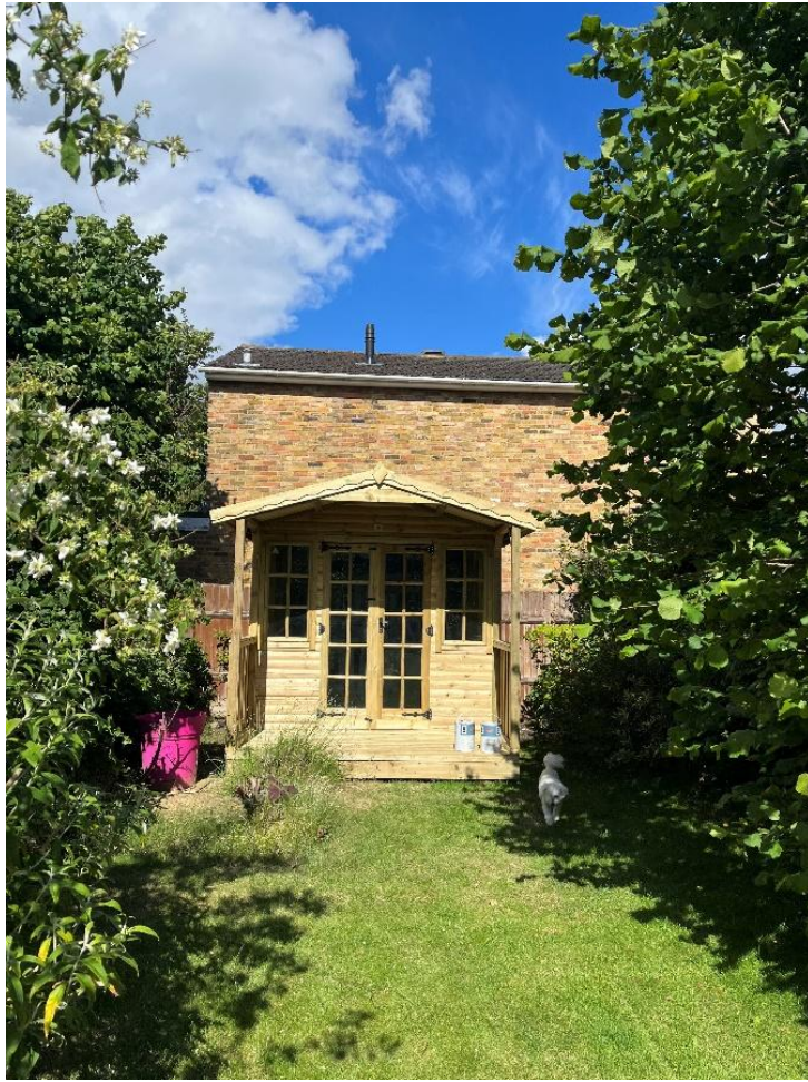
Figure 2 – view of outbuilding at 128 Ship Lane
